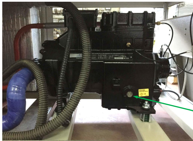
Figure 5-6. Compressor (rear view)
