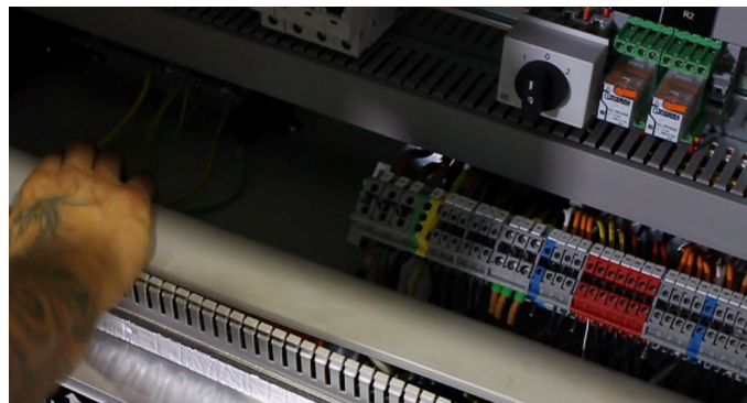
Figure 4-7. Replacing wire channel cover
